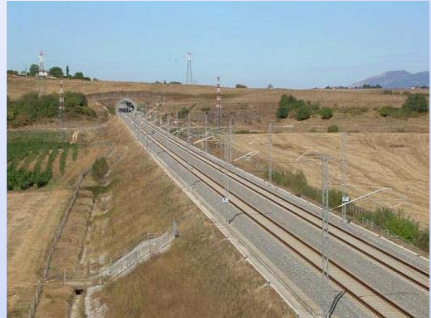
Example of railway on embankment Rome - Naples
