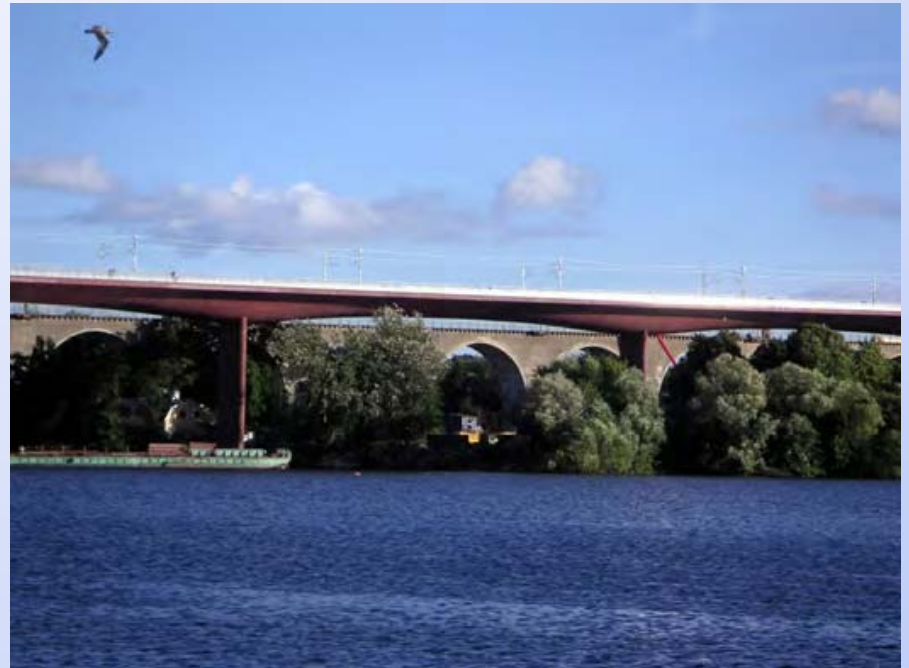
Arsta viaduct (Arup)
