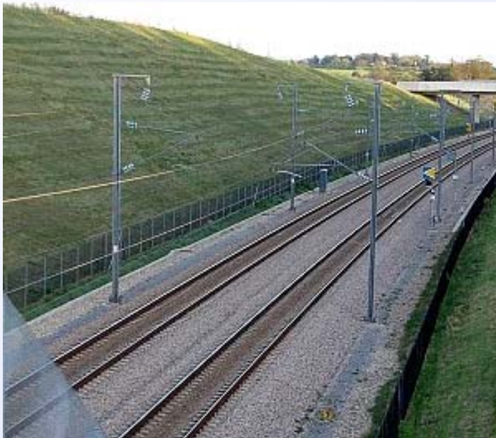
Example of railway in cutting High Speed 1
